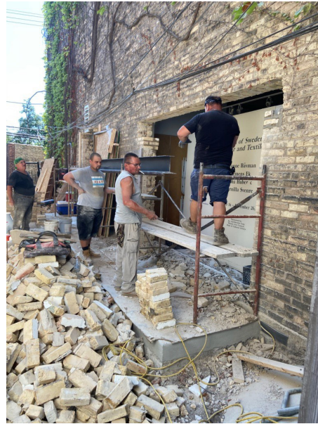
Photo: Work on the opening from the Gallery to the garden.
